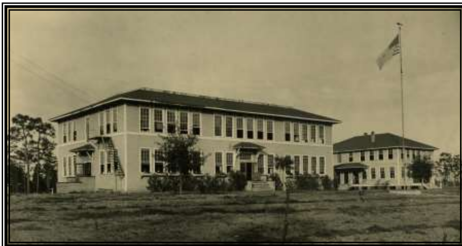
Kiln High School Kiln, MS
