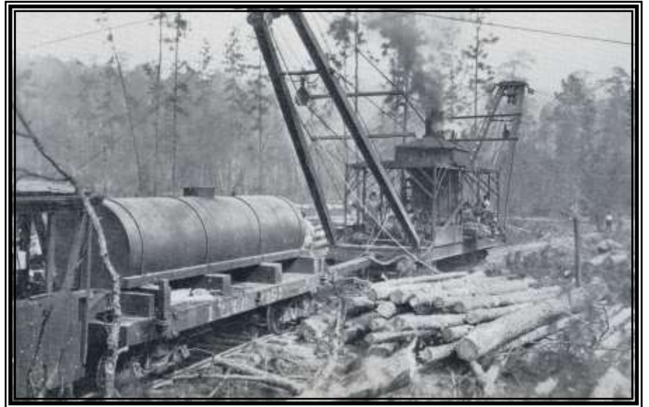
This Clyde two-line skidder is a good example of the ones used in Hancock County by the timber industry in the early nineteen hundreds.
