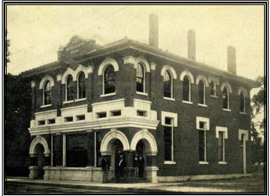
Merchants Bank Formerly located at 205 South Beach Blvd., Bay St. Louis, Mississippi Building destroyed by Hurricane Katrina, 2005
