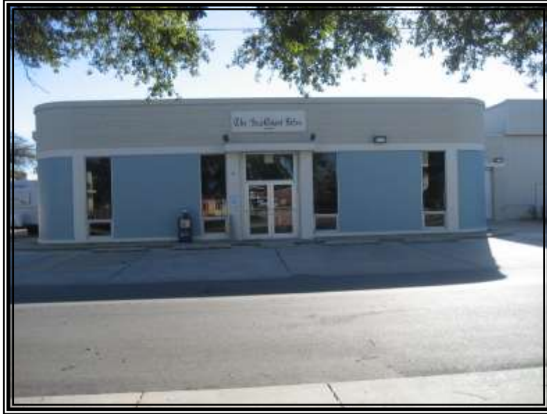
This is the current home of the Sea Coast Echo at 124 Court Street in Bay St. Louis.
