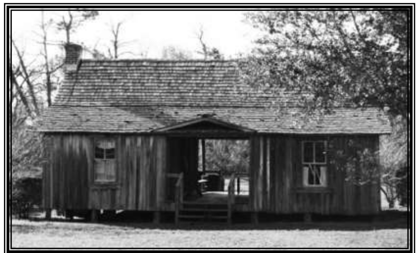
This dog trot house is quite similar to the ones built by early settlers in Hancock County. One which older residents may remember was the Koch house in the Logtown area before additions were added and before it was moved because it was in the buffer zone of the Stennis Space Center.
