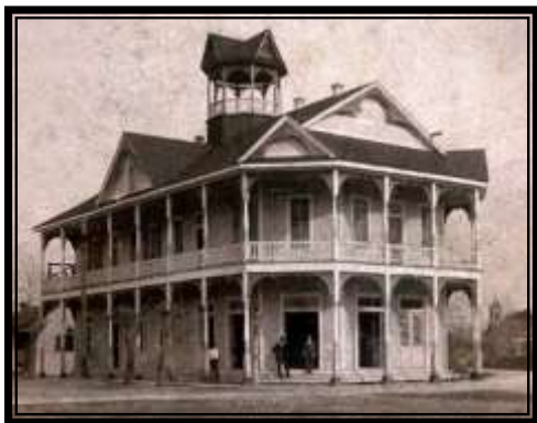
This is the Gilmore Hotel located across Railroad Street (Blaze Ave.) from the train depot.
