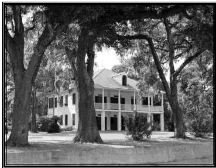
Later named Elmwood , the manor house of the Cowand Plantation stood at 900 North Beach Blvd. in Bay St. Louis. When it was built in 1803, it stood on forest land fronting the western edge of the Bay of St. Louis, many years later enveloped by the City of Bay St. Louis. It was completely destroyed by Hurricane Katrina in August 2005.
