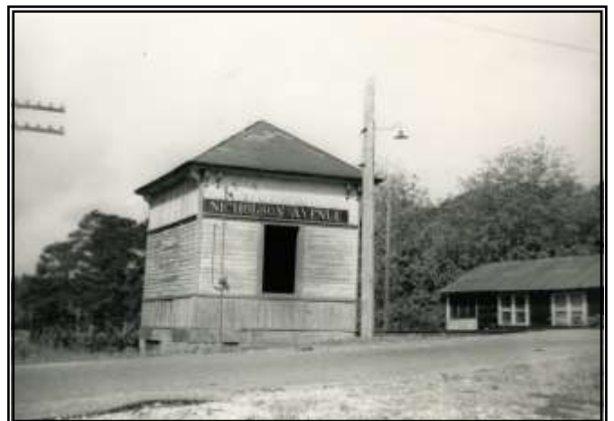
The Nicholson Avenue depot
