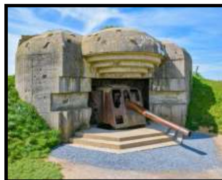
A pillbox is a type of blockhouse, or concrete dug-in guard post normally equipped with loopholes through which to fire weapons.
