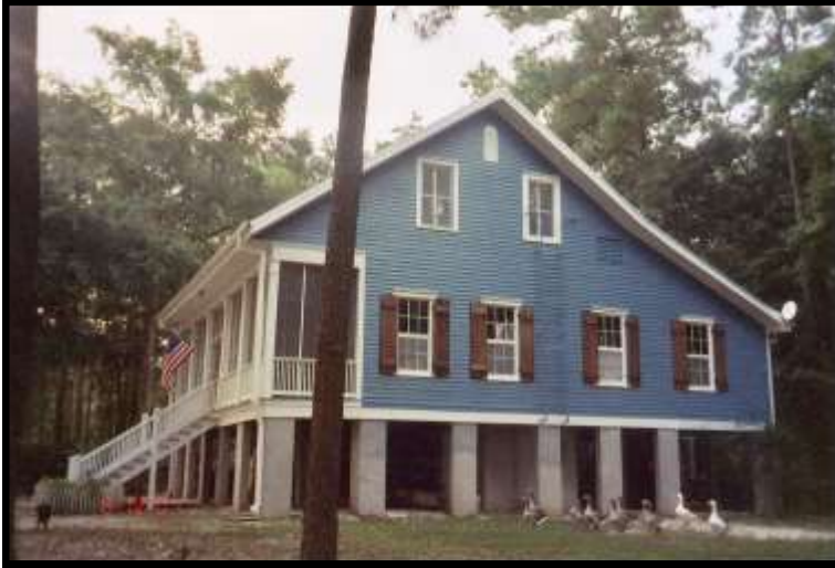
The renovated Vaughn house, seen from this angle, demonstrates the classic features of a Creole cottage. The house is raised on piers, has a tall, steep roof, and a cut-away gallery in front. The front of the cottage was rotated to face the Pearl River instead of the Gin Road, when moved in 1972.
