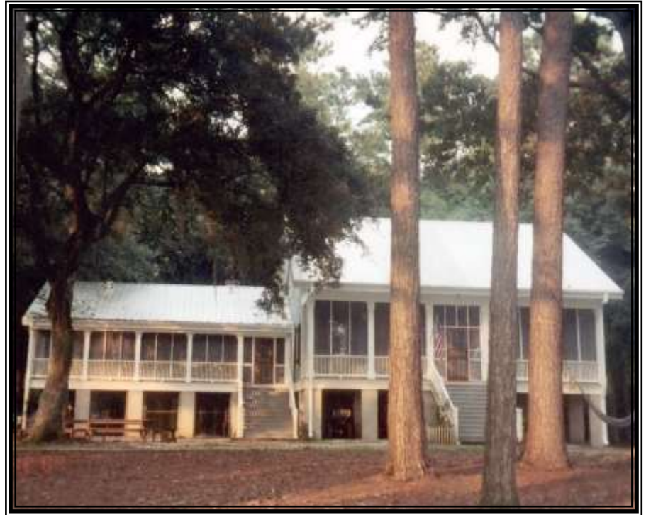
The Vaughn house in Pearlinton was a vintage Creole Cottage. The building in this photo shows the renovations made by the Viguere family. The original Creole cottage is to the reader's right and there is an addition to the left made by the Viguere family.
