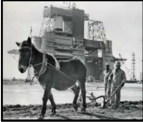
A mule was important in the construction of an infrastructure pipeline during the building of the Stennis Space Center.
